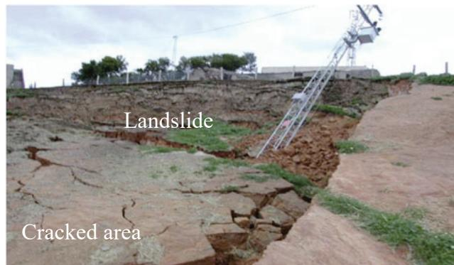
Figure 2. Damage of structures induced by desiccation cracks.
